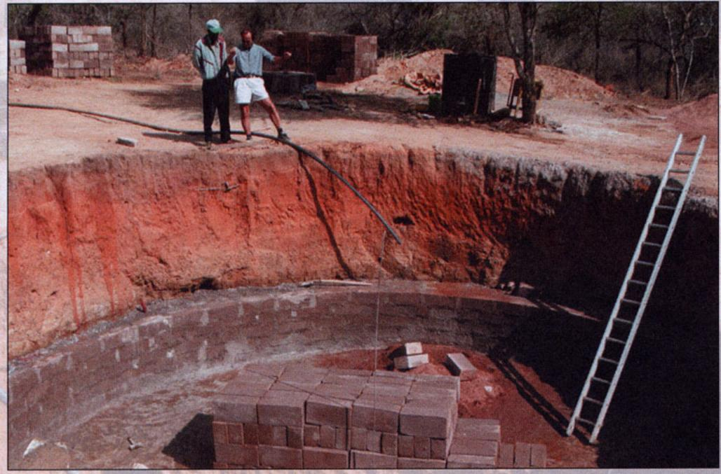
water for 18 months, since it was completed, and is holding up well. Tony felt that a further emergency water source was necessary, water being the perennial problem in Mkomazi. This new storage tank has the capacity for 75,000 gallons (341,250 litres). Filtration and treatment systems are also being installed. *Tanga Cement*, through Basil Hersov, agreed to donate 500 bags of cement for this project, which was a fantastic step forward and for which we are very grateful.
