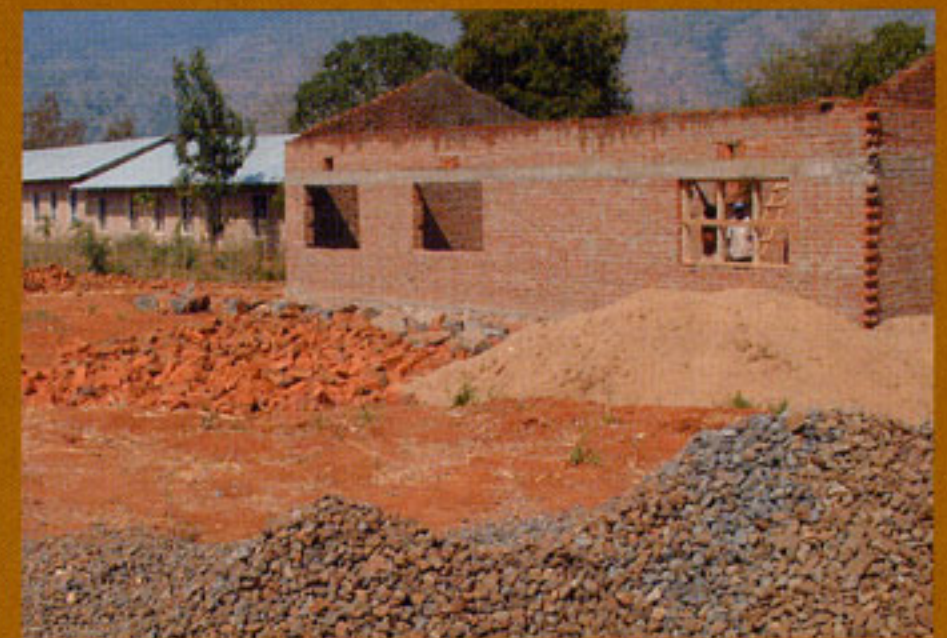
Above: Kisiwani Secondary School science laboratory under construction.
