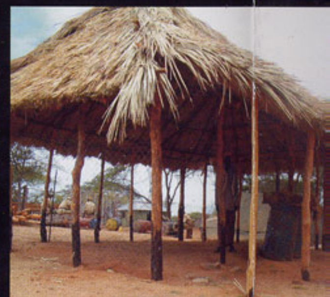
Mess hut under construction, Kampi
