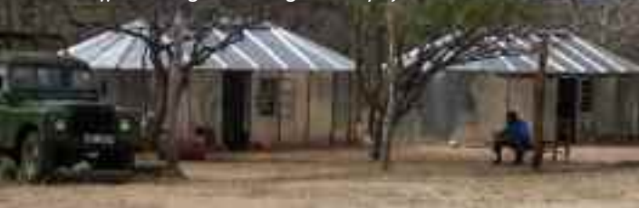
New staff and ranger housing at Kampi ya Simba
