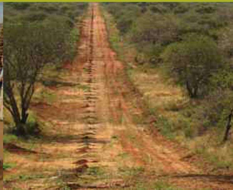
Fence post holes dug by hand for the Mkomazi Rhino Sanctuary Extension
