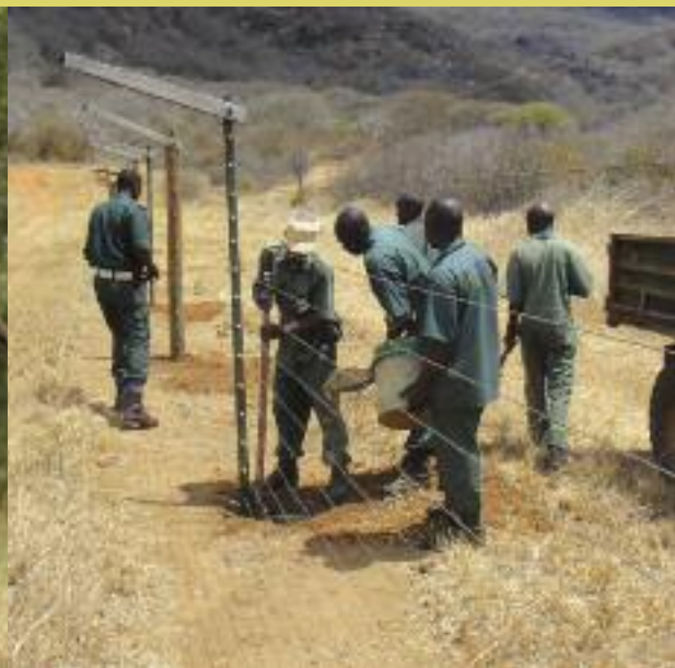
Rhino Sanctuary fence repair team at work
