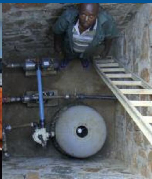
Eliyudi installing new water pumping and filtration system
