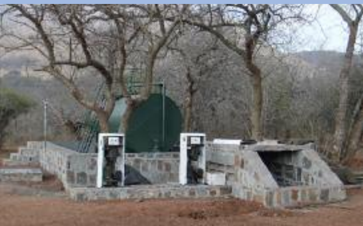
Fuel storage tanks completed and pumps awaiting calibration by Puma Energy
