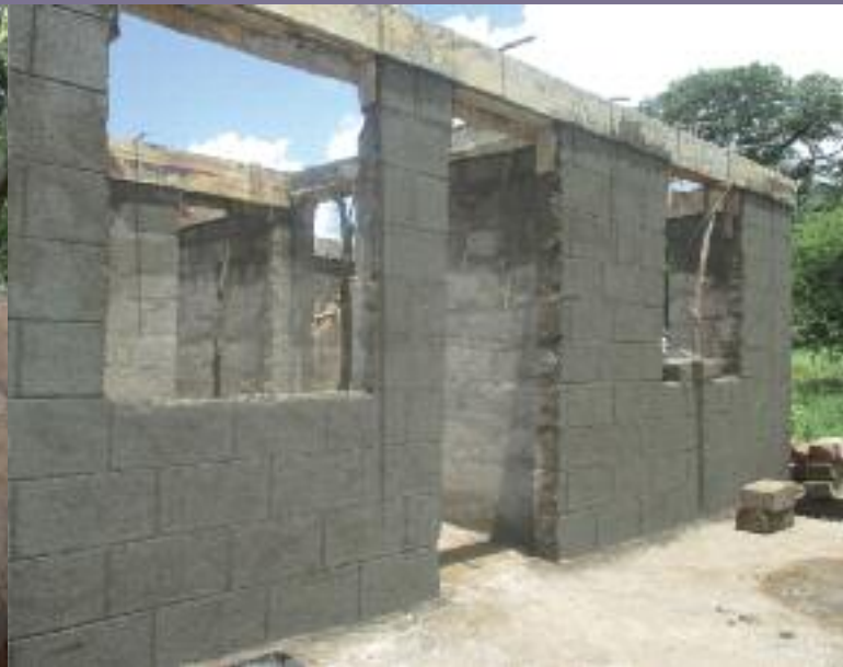
VTC administration office being built
