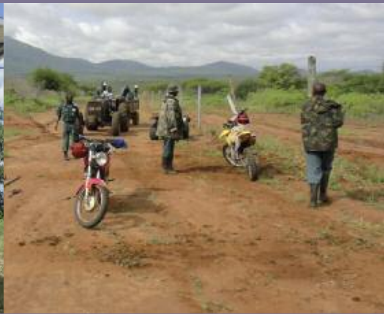
Mkomazi Rhino Sanctuary fence repair – a daily undertaking
