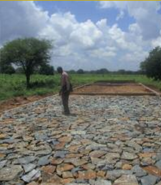
Foundations being laid for classrooms at the Gonja VTC
