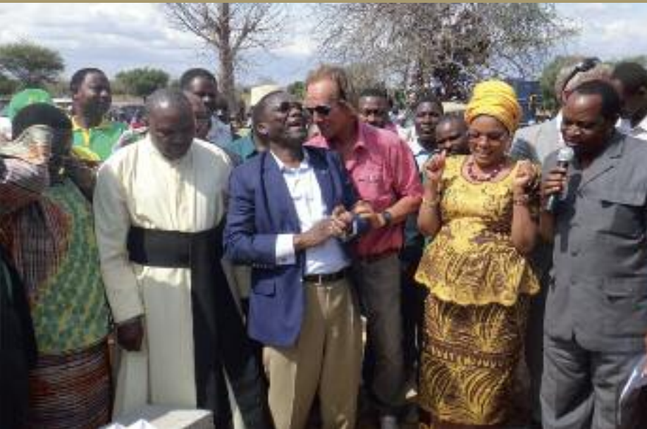
With the Prime Minister of Tanzania, Hon. Mizengo Pinda, at the laying of the foundation stone for the vocational training centre. From left: Vicar General Everesti, the Prime Minister, Anne Kilango MP and DC Herman Kapufi
