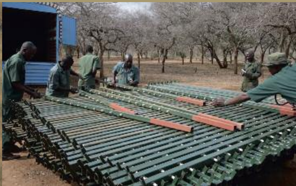
Steel fence posts delivered and stacked for rhino sanctuary repairs
