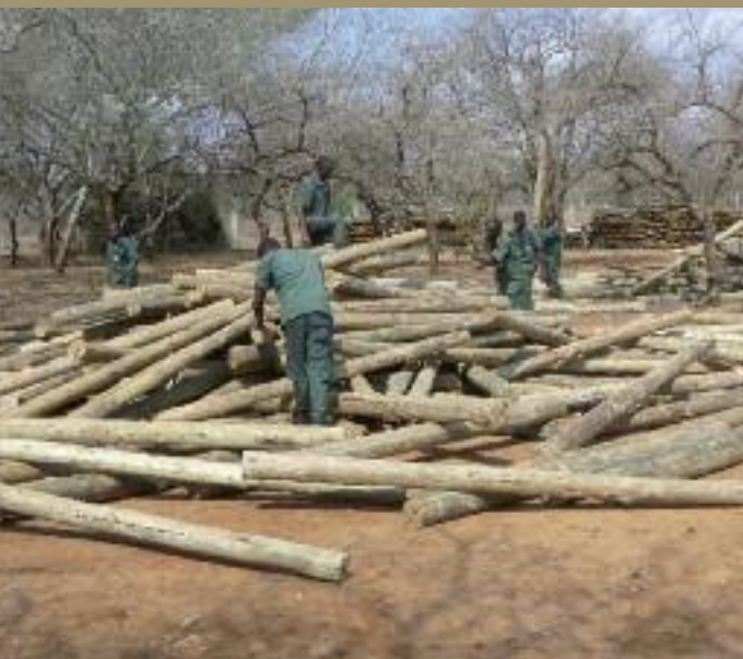
New fence posts are delivered and sorted
