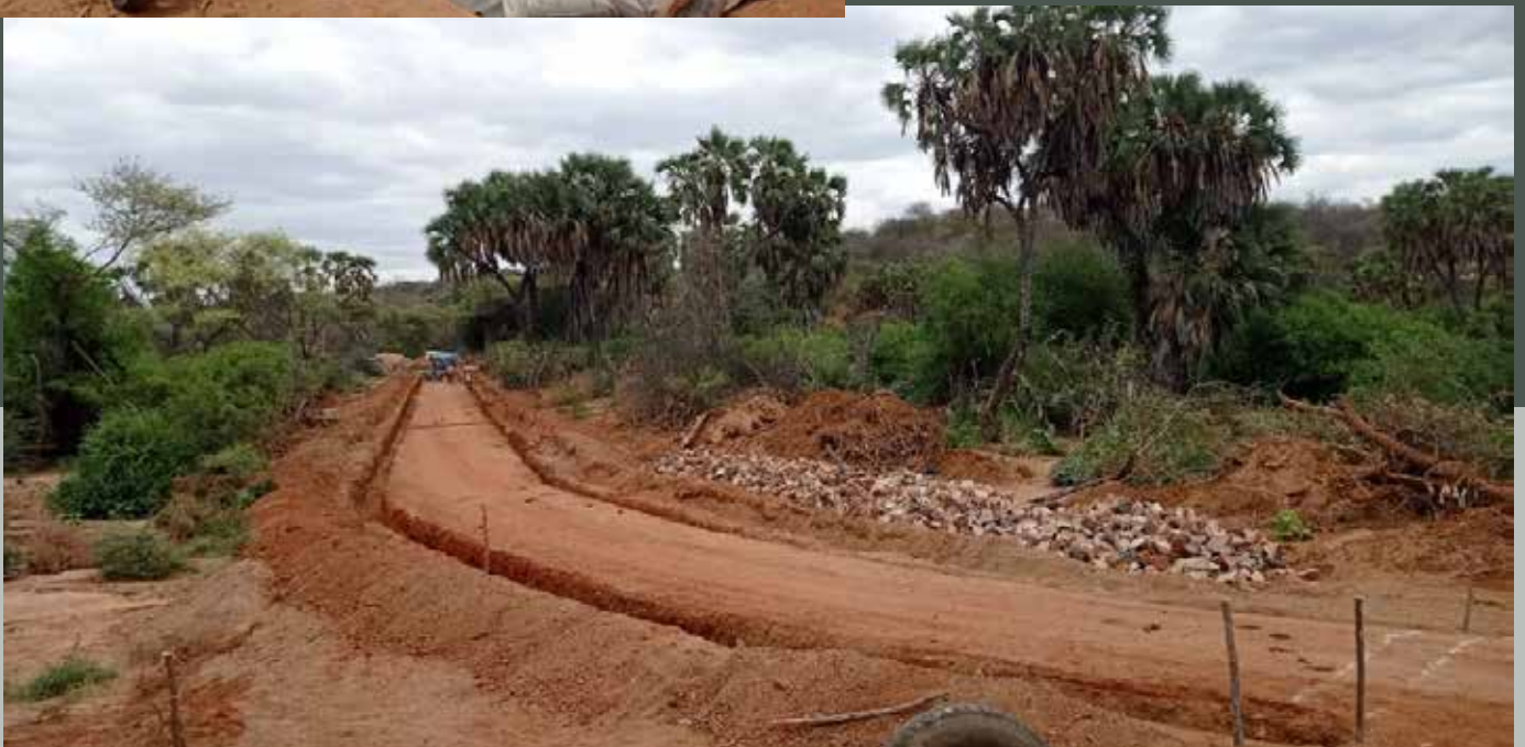
KWS drift bridge being put in place at Kyethoni lugga (water channel)
