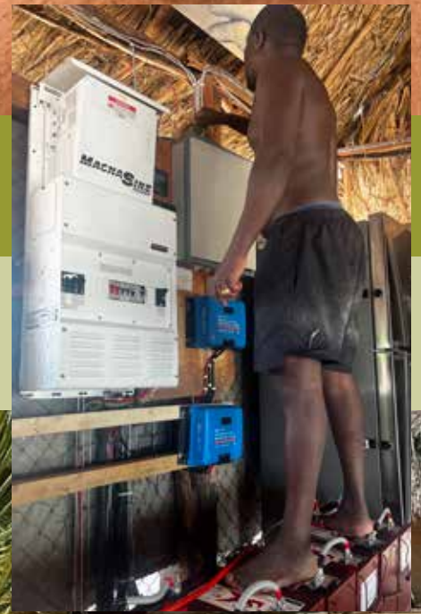
Vincent installing solar equipment
