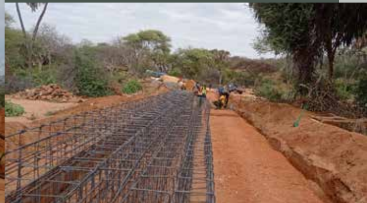
KWS drift bridge being put in place at Kyethoni lugga (water channel)
