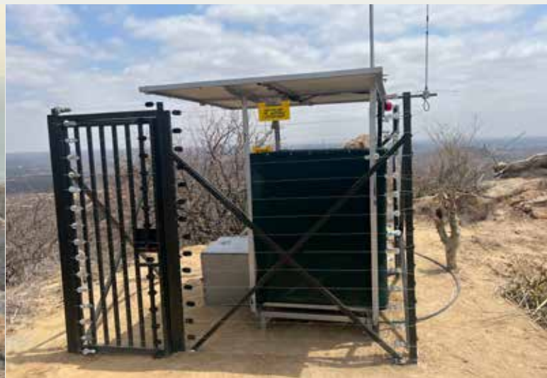
Radio repeater and solar powered electric fencing
