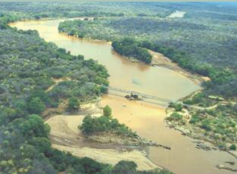
Bridge over the Tana River linking Kora and Meru National Parks
