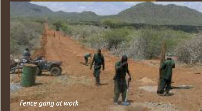
New fencing construction - strainer posts go in
