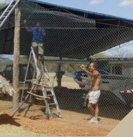
re-fabric'd (hessian, chicken wire, cement) and the structure roofing was redone with locally cut poles. Piping and electrical wires that had been chewed by rats were repaired, water systems upgraded
