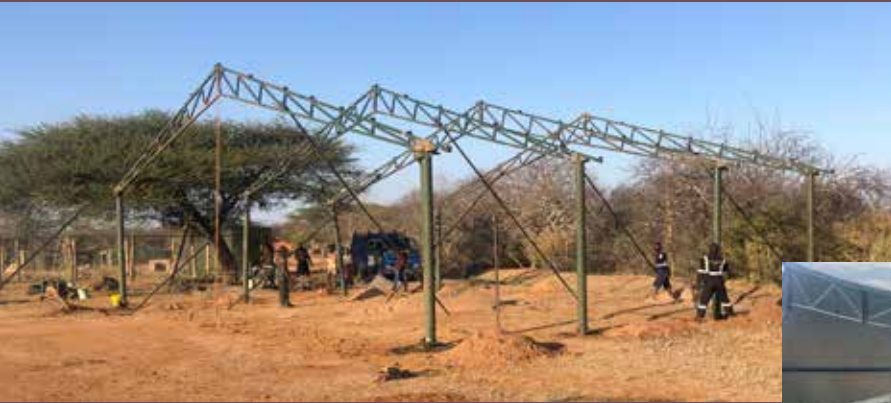
Hangars go up
