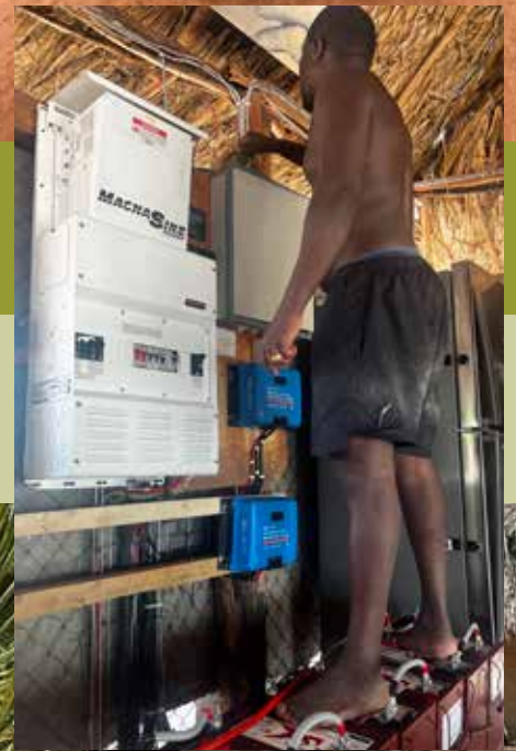
Vincent installing solar equipment
